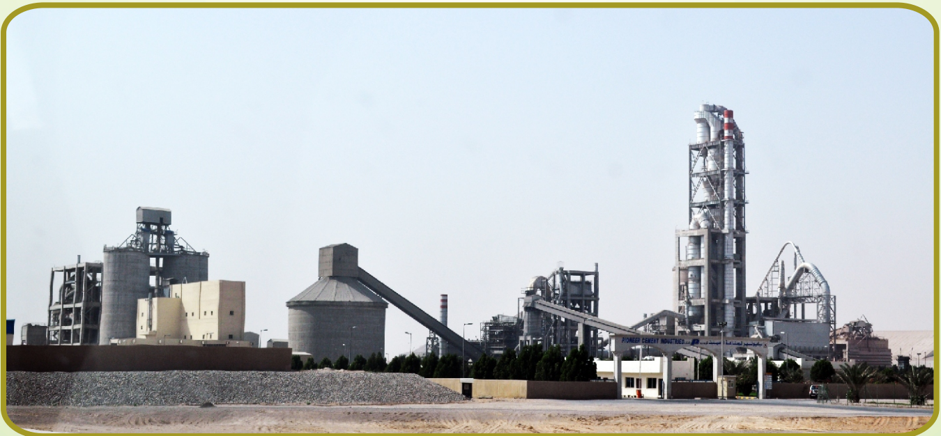
PIONEER CEMENT INDUSTRIES LLC, UAE
