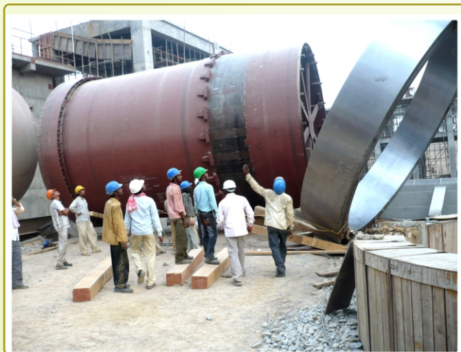
Kiln Erection at Jaypee Cements Dhala, Uthar Pradesh
