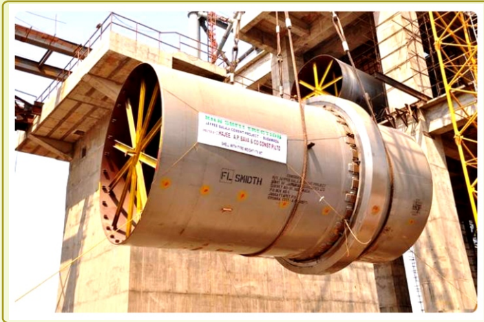
Kiln Erection at JP Balaji Cements Jaggayapet, A.P
