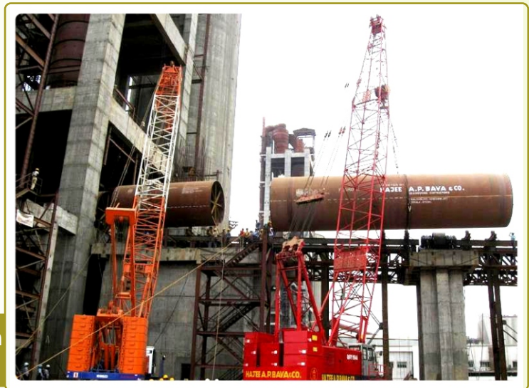
Kiln Shell Erection CCCL Ariyallur, TN
