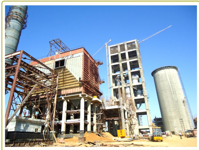
Erection of ESP at ABG Cements Kutch, Gujarat
