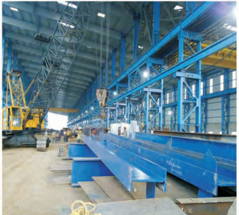
Fabrication At BWP
