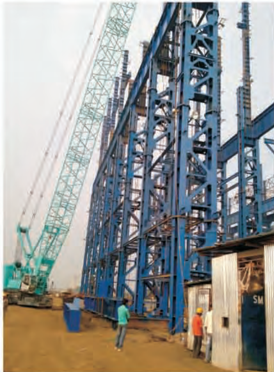
Erection Of Sms Column By 250 Ton Crane
