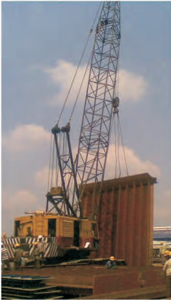
LDP-Fab of bunker 95 ton
