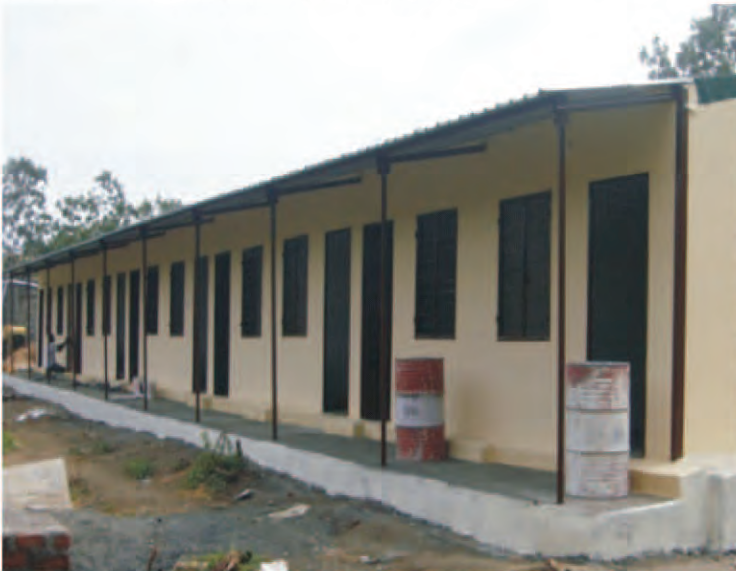
Staff Quarters Aerocon Building UTCL Rajasree site
