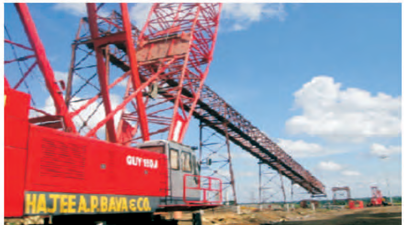
Cement Ball Mill Erection at CCCL Kallur
