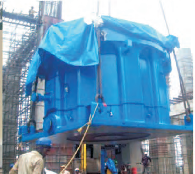
Erection of Vertical Gear Box at BCCL Kadapa
