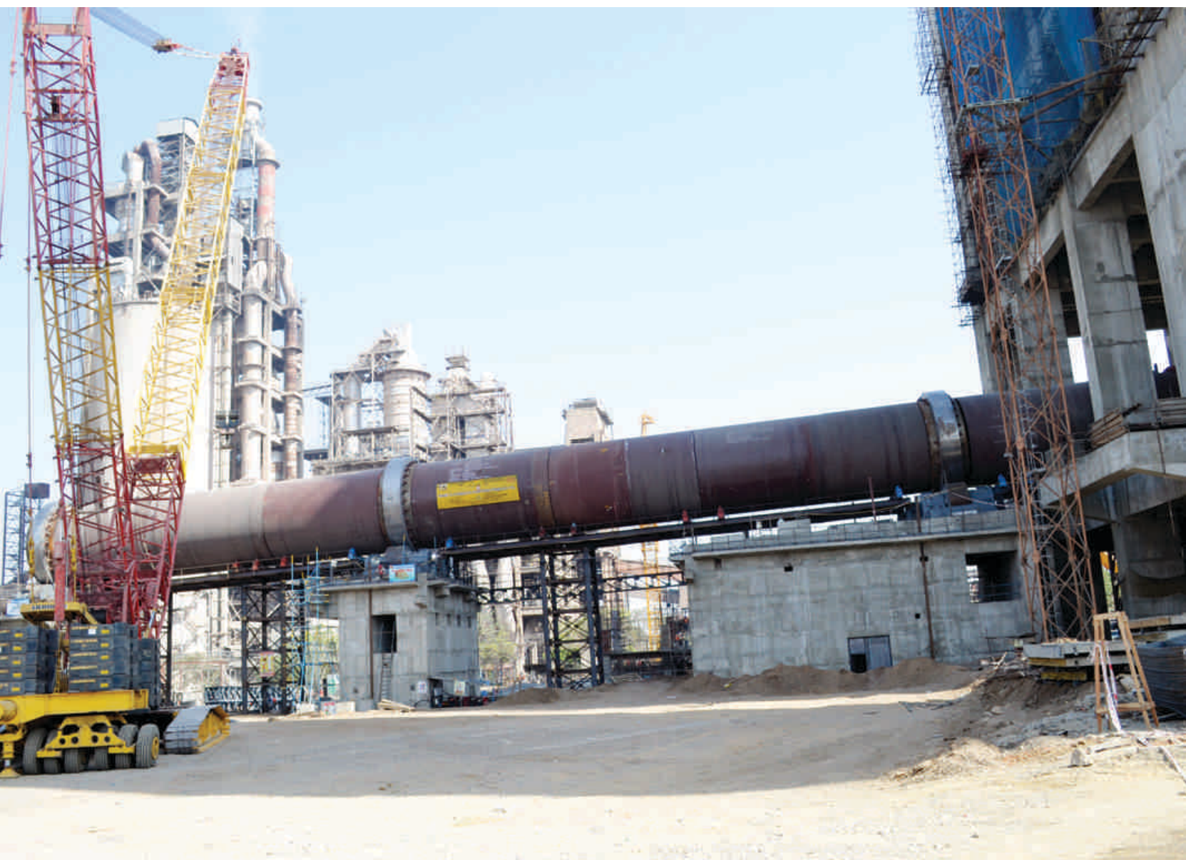
Kiln Erection at Ultratech Cements Rawan
