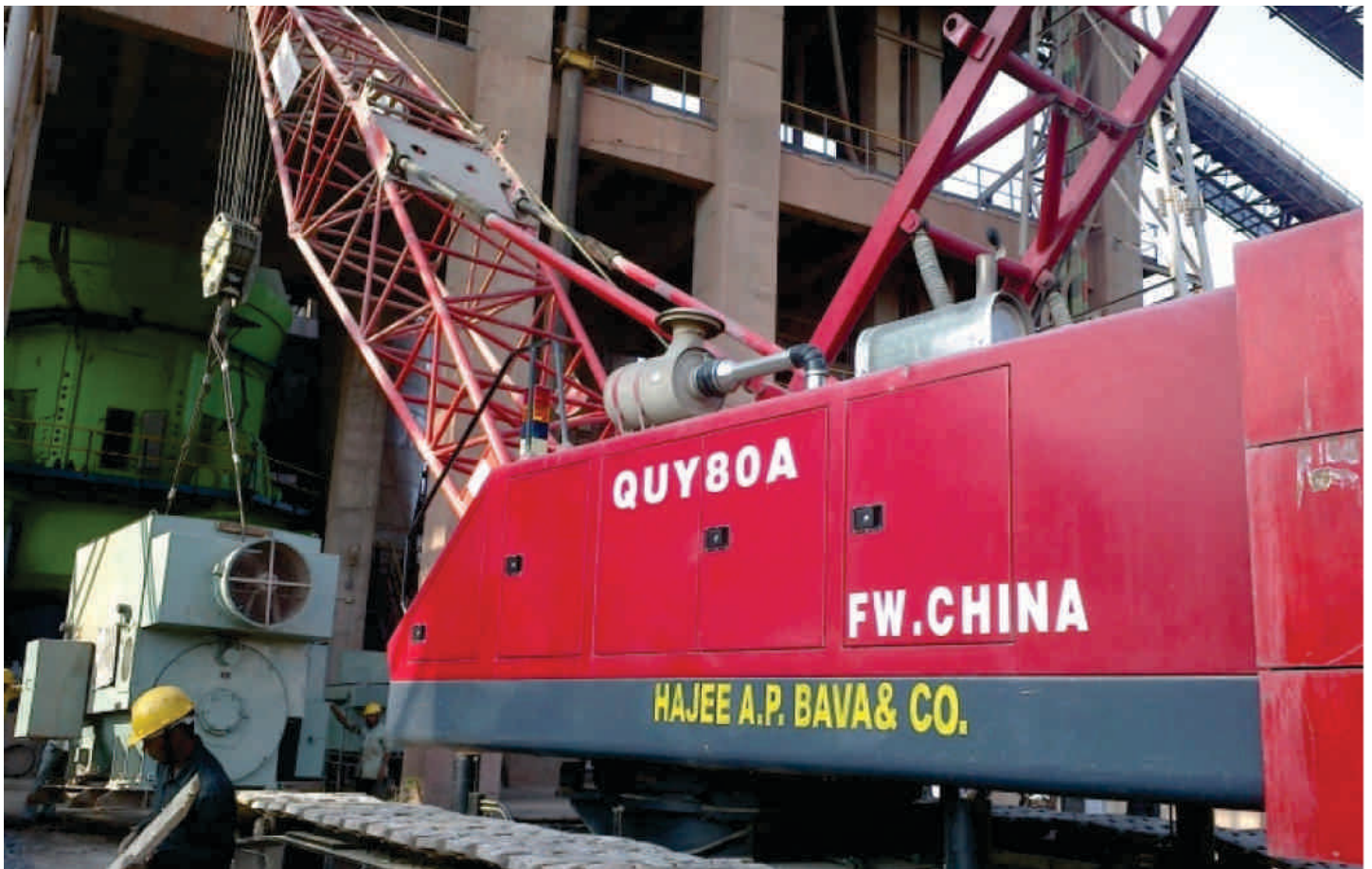
Erection of Machinery at BCCL, Kadapa
