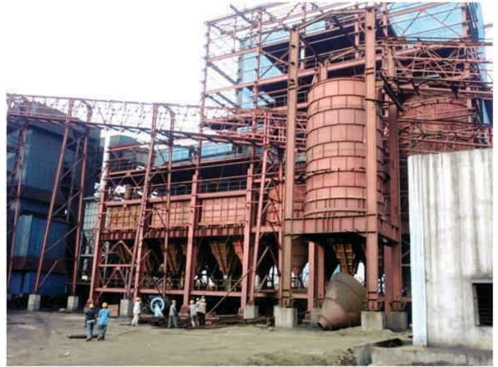
VIEW OF SUPER SMELTER SITE, WB
