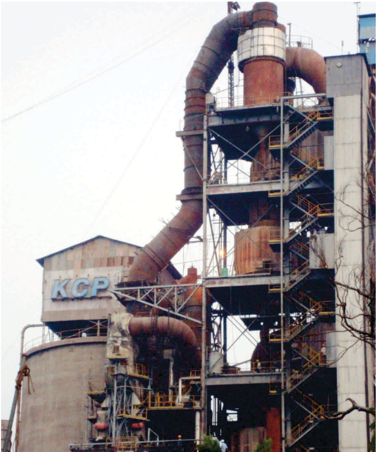
KCP RAMAKRISHNA CEMENTS(SHUTDOWN WORK)
