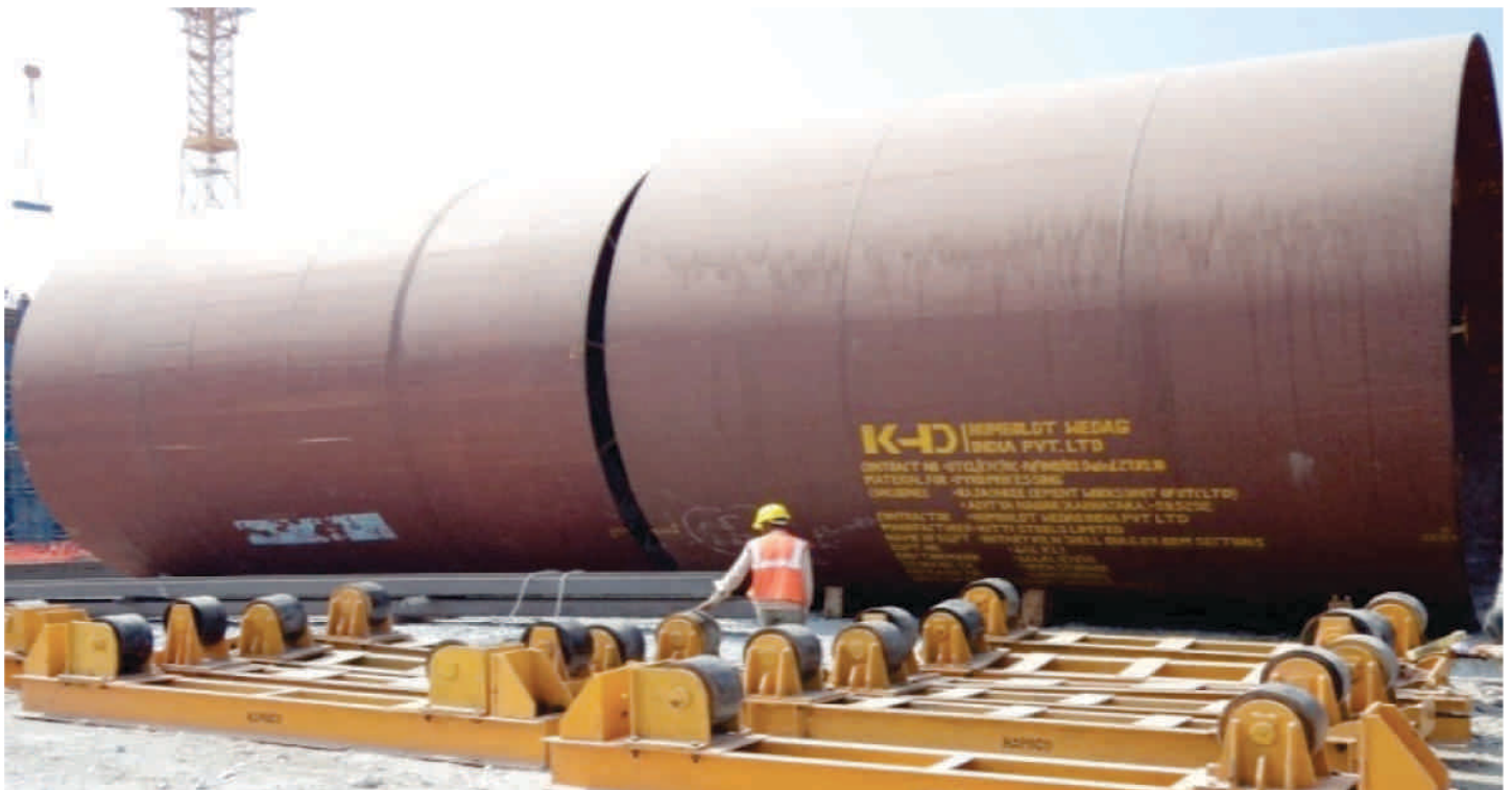
KILN SHELL GROUND ASSEMBLY NEAR KILN PIER, At UTCL Rajasree cements
