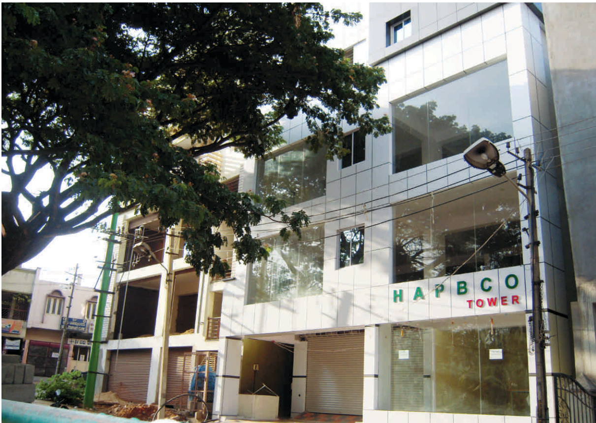
HAPBCO Tower at Bengaluru
