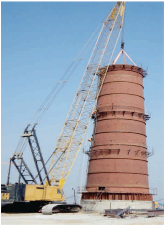
ERECTION OF COOLER STACK UTCL Rajasree cements
