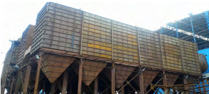
Volume of bag house 4400000 Am 3 /hrs and India's largest bag-house in steel industry
