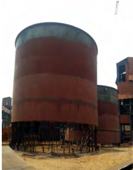
Slurry Tank (14 mtr dia x 21 mtr height ) Fab&Erec Through hydraulic system AT JSPL ( BARBIL ) II PH EXPANSION PELLET PLANT PROJECT
