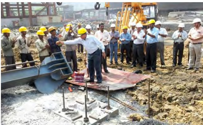
Mr.G.P GUPTA, GM-Projects, Mr.B.M Singh, GM-Quality (M/s. Prayagaraj Thermal Power Plant (Jaypee)), Guest of Honour in our Work resumption Ceremony of Jaypee 660 X 3 MW Power Plant on 25.12.12
