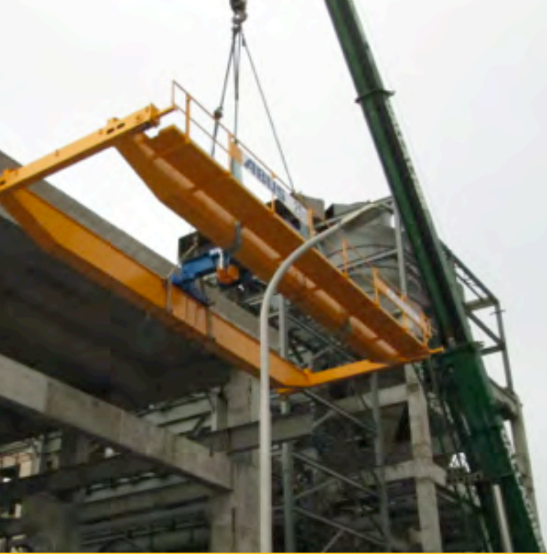
EOT Crane Erection at ABG STAR
