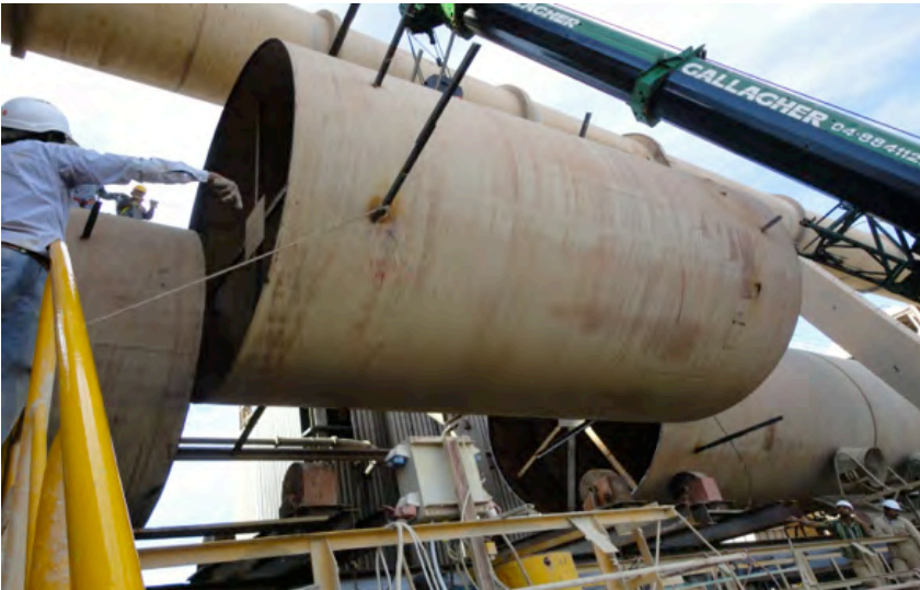
Kiln shell replacement
