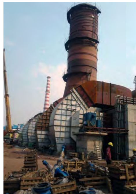
MONNET ISPATH & ENERGY LTD-AIR COOLER DUCT ERECTION -6100 mm Dia and TOTAL LENTH OF DUCT 600 mtr
