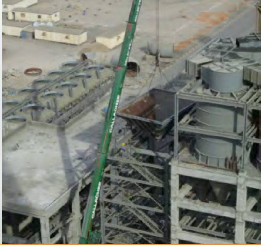
Hopper Erection at WHRS-Star
