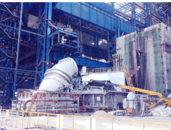
India's biggest 250tons electric arc furnace
