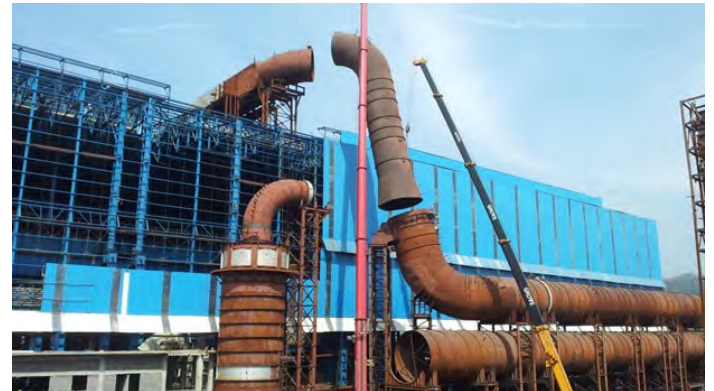
MONNET ISPATH & ENERGY LTD-AIR COOLER DUCT ERECTION -6100 mm Dia and TOTAL LENTH OF DUCT 600 mtr
