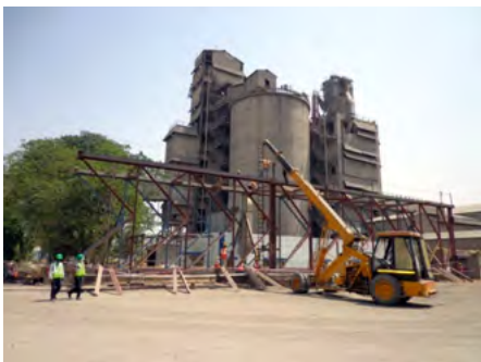
Slurry Tank (14 mtr dia x 21 mtr height ) Fab&Erec Through hydraulic system AT JSPL ( BARBIL ) II PH EXPANSION PELLET PLANT PROJECT
