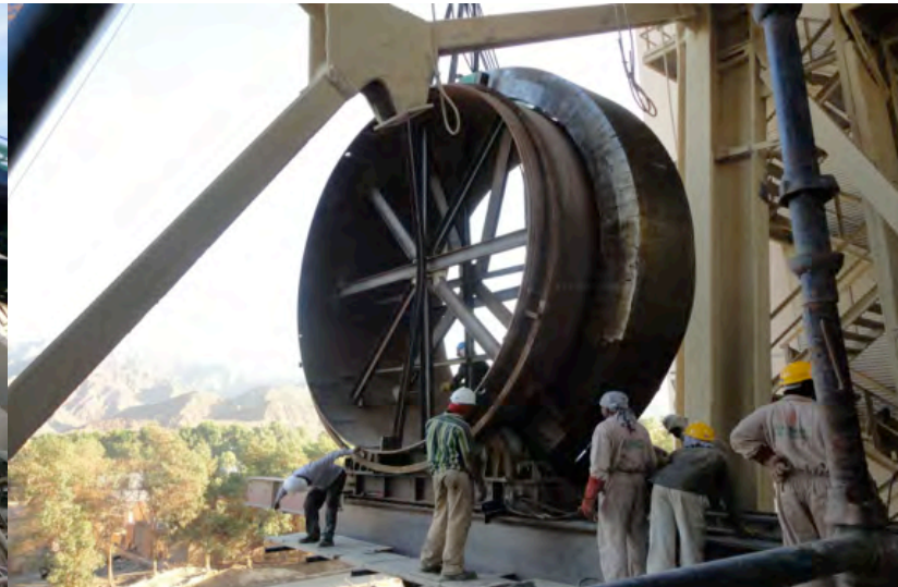
Tyre Assembled in new shell
