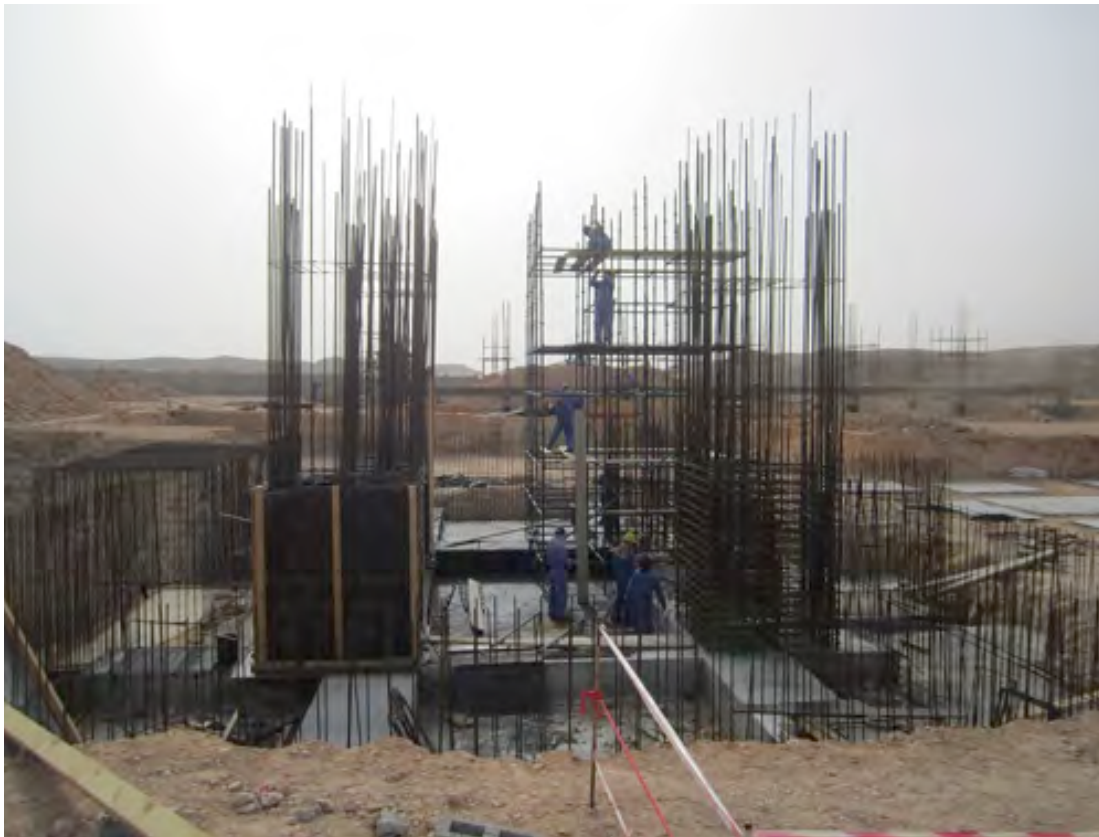
Kiln Foundation & building
