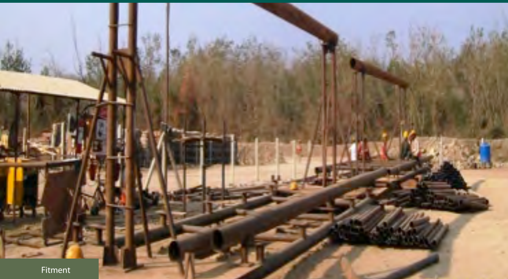
Pipe Conveyor structure erection
